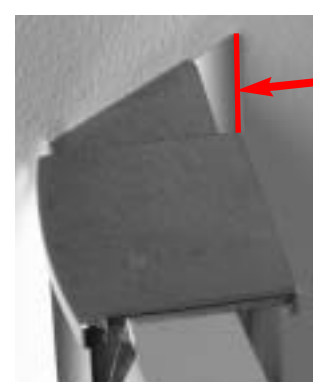
16 Press on cover caps V2106L/R or V2107L/R to wall & V2101L/R to frame profiles.
