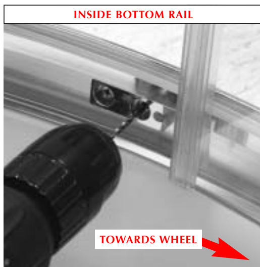
13 Screw the back hole of the LONG roller stop V6105 to the pre-drilled hole on the inside of the bottom profile. Drill through the front hole and screw. Insert cover caps V2111.
